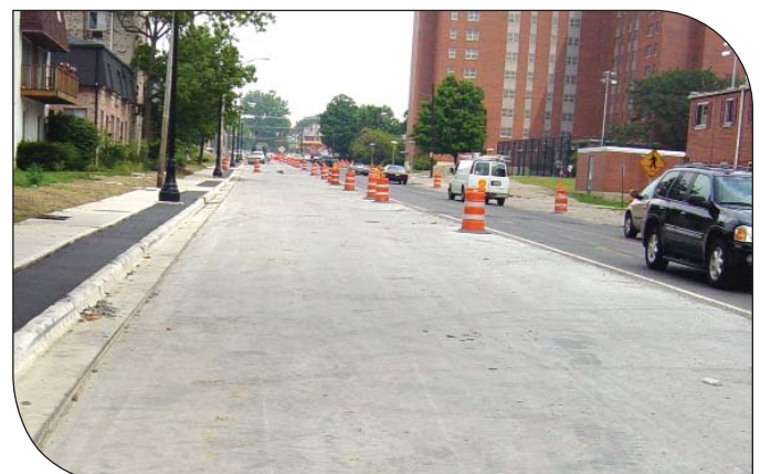
RCC can be constructed with minimum disruption of traffic.
