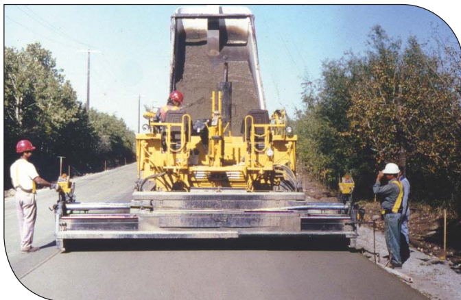
Road widening made easy with roller-compacted concrete.
