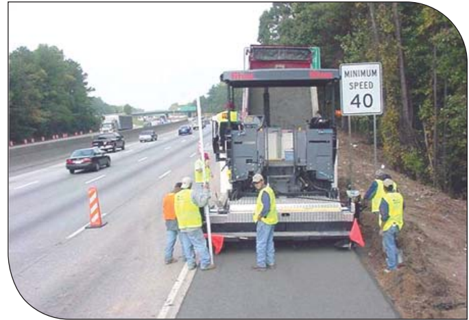
RCC was used to reconstruct shoulders along I-285 in Atlanta.
